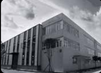
Production base in Pujiang, Sichuan
