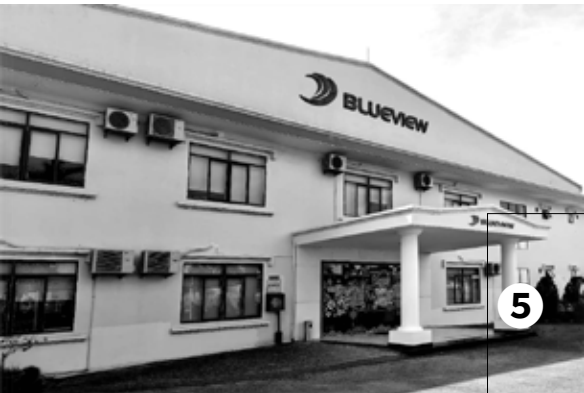
Production base in Hai Phong, Vietnam
